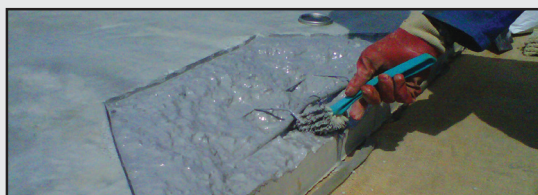
BONDING FRESH CONCRETE TO EXISTING CONCRETE
